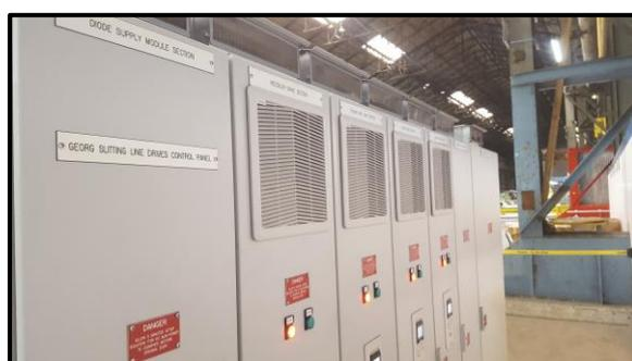
**Caption:** An AC multidrive system applied to Tata Steel’s slitting line has eliminated stoppages, increased production and cut costs.
